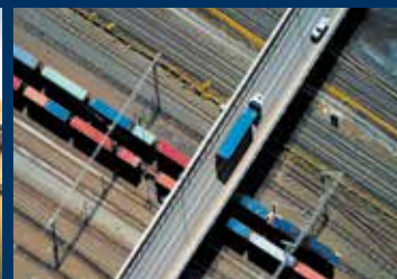
Enfield Intermodal Logistics Centre
