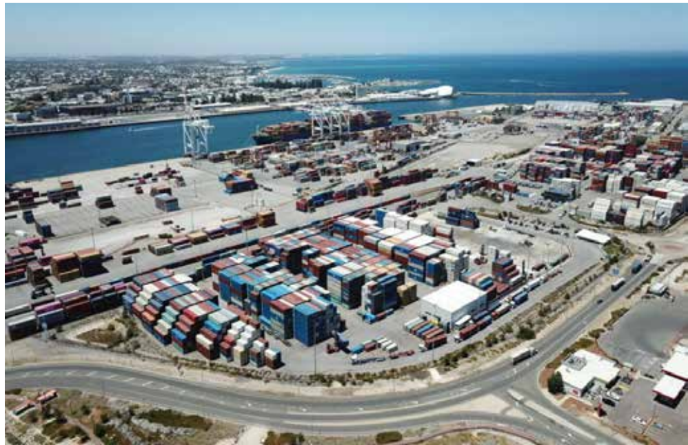
TYNE ACFS Fremantle container park was designed around efficiency
