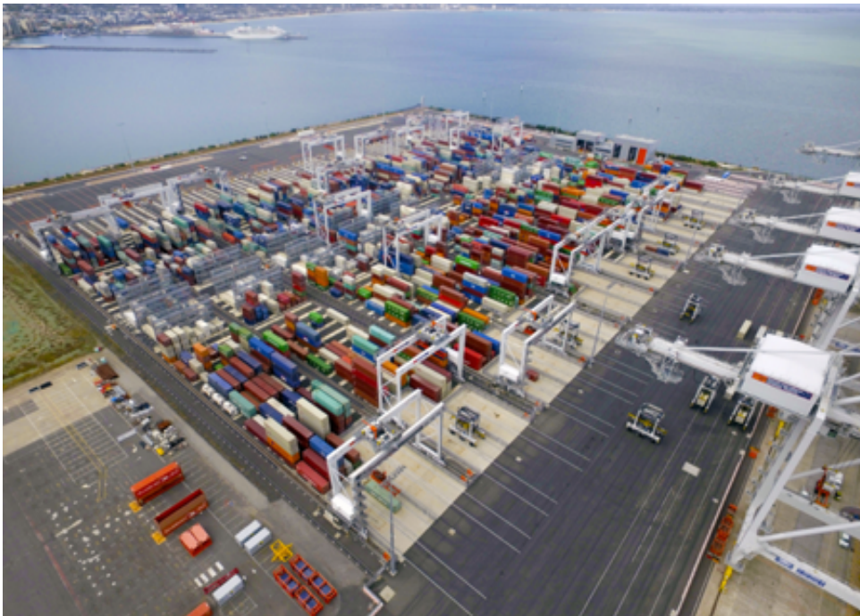
Victoria International Container Terminal (VICT) – Australia's first fully automated container terminal at Webb Dock East, Port Melbourne.
